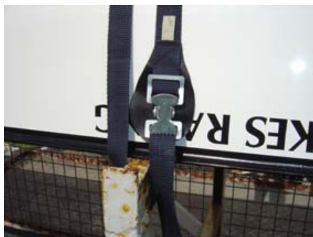
Too thin Wrong!
